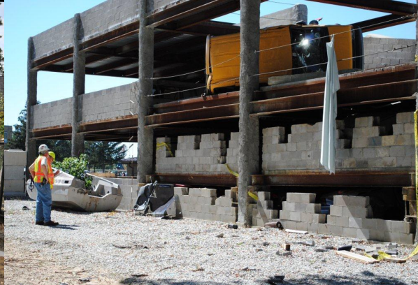
I-BEAM evaluates the safety of a parking garage building.
