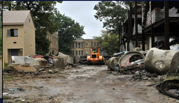
INDOT participated by deploying debris removal teams
